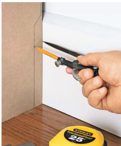
Cut the template to match the project part to be scribed. Set it in place, plumb and level it, and scribe it just like the project part itself.
