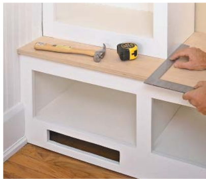
Use a framing square to make sure each tall case is positioned properly before scribing it and before installing it.
