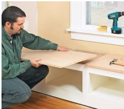
Each seat panel gets trimmed to fit the wall on the back and outside end. The panels should meet tightly at the center.
